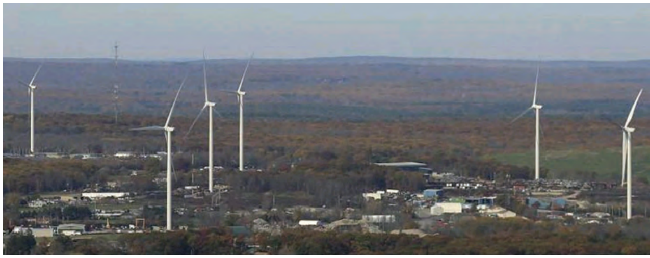
JOHNSTON WIND: Green Development built and operates the Johnston Wind Project, along Plainfield Pike and Shun Turnpike in Johnston. Johnston Wind consists of seven 3-MW wind turbines completed in 2018 and operational since December 2018. (Photo courtesy Green Development)
